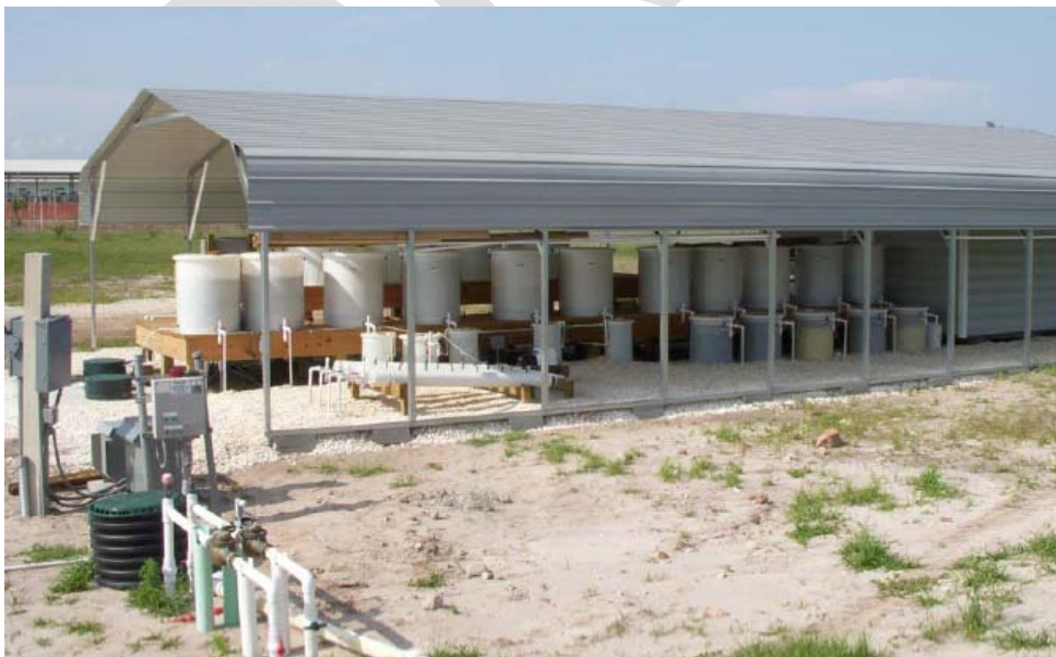
Figure 2. Test facility constructed at the University of Florida's Gulf Coast Research & Education Center.
